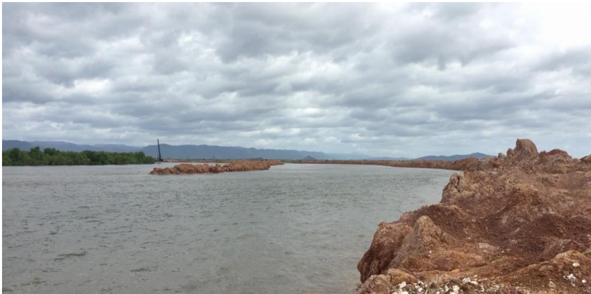
Figure 8: Image of the dredged river channel taken from the top of one embankment. Koh Samao is visible on the left. The photo looks north towards the proposed pier location.
