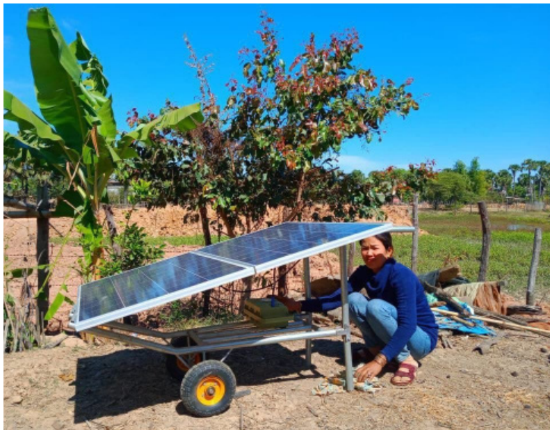
Sreymich was checking the solar water pump before she used.
